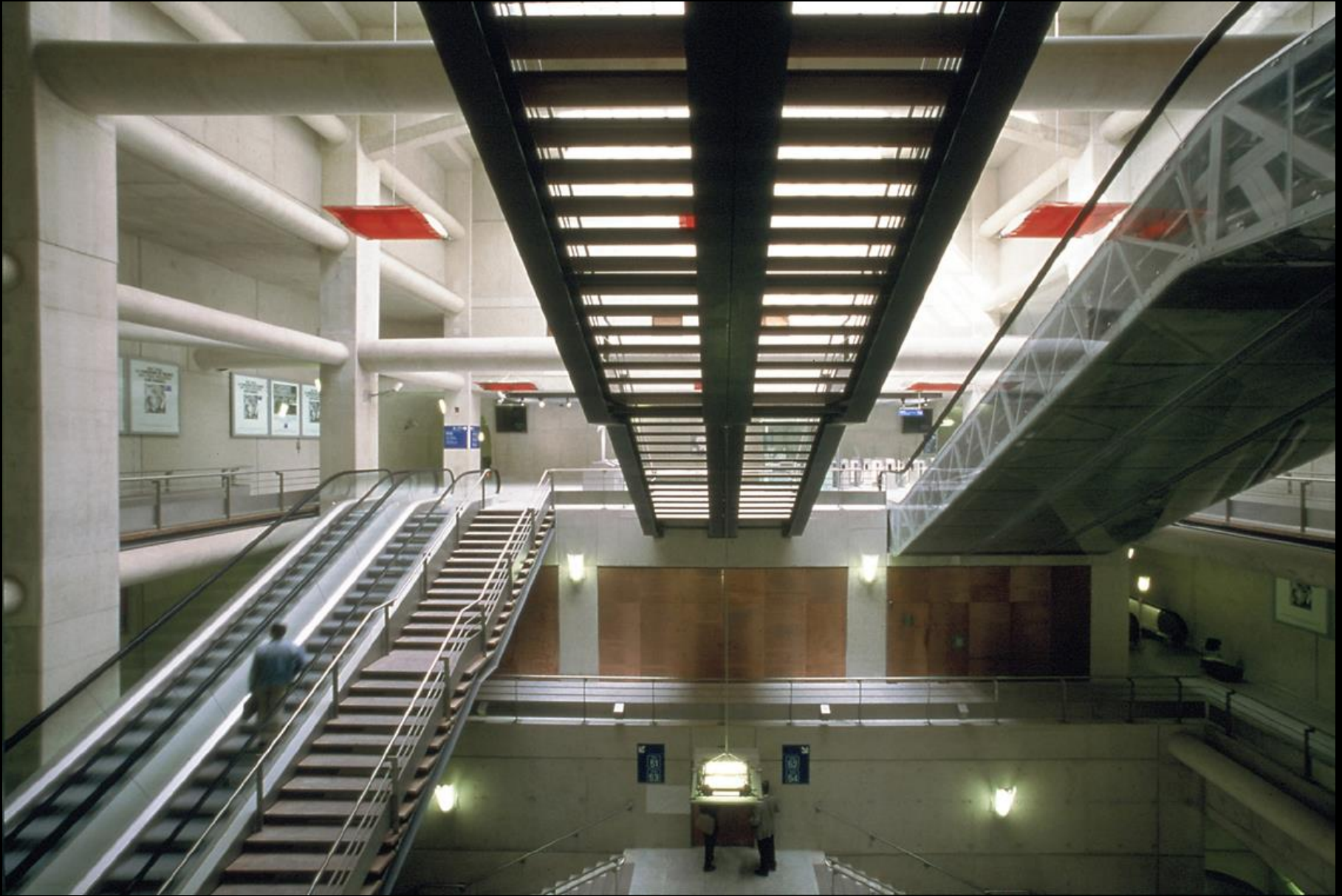
Passengers are constantly aware of exactly where they are within the well lit station complex - Gare de Magenta RER E, regional express train station, Paris
