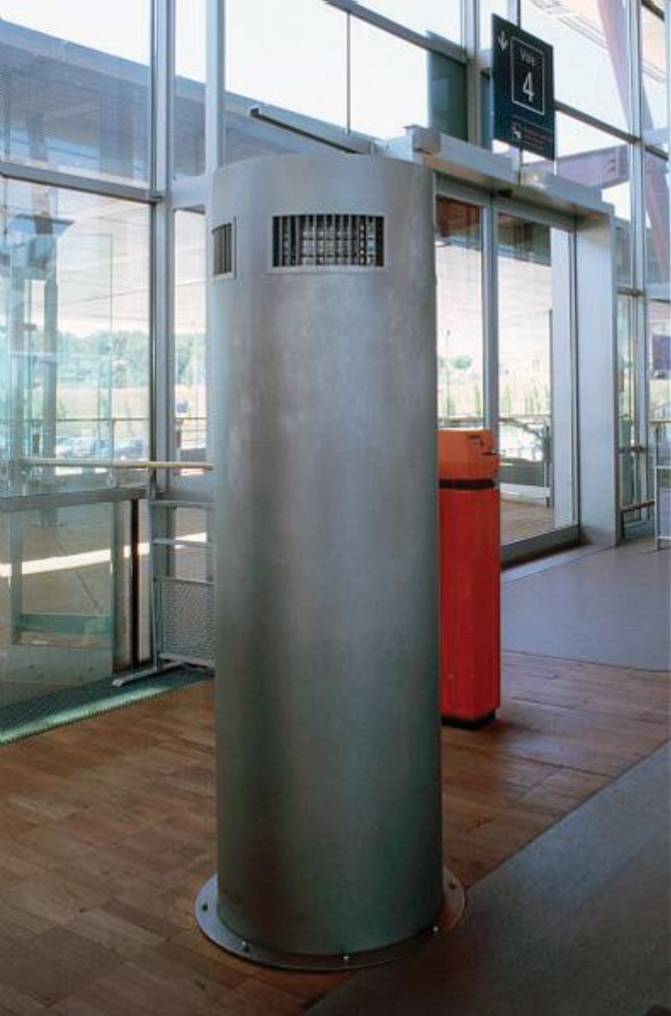
Air conditioned outlet device Valence high speed train station, France.
