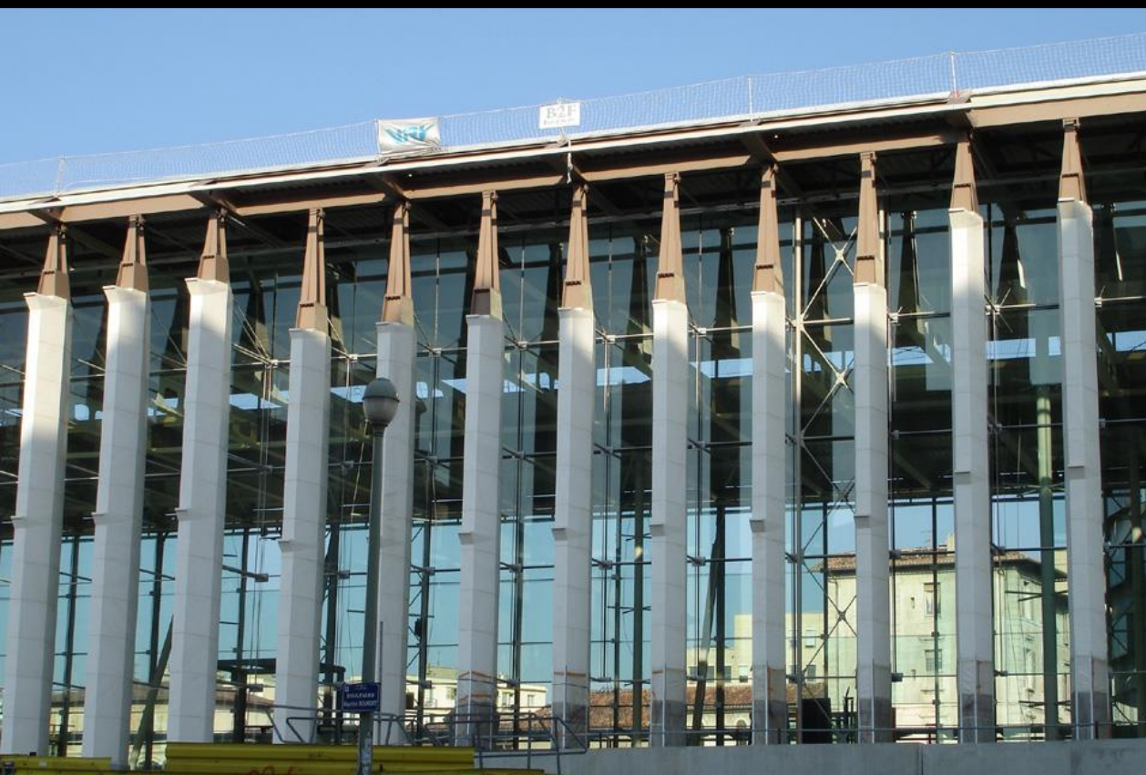
Local stone and innovative technique : The pre-stressed pillars
