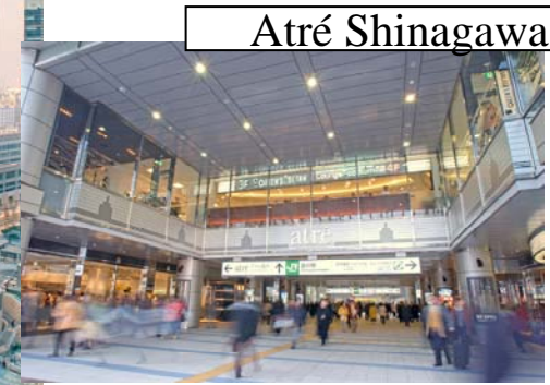
JR Shinagawa East Building
